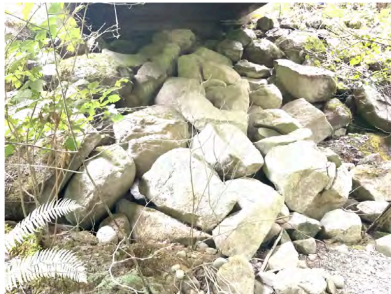
Left Bank Abutment when facing downstream
