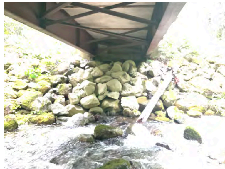
Right Bank Abutment when facing downstream
